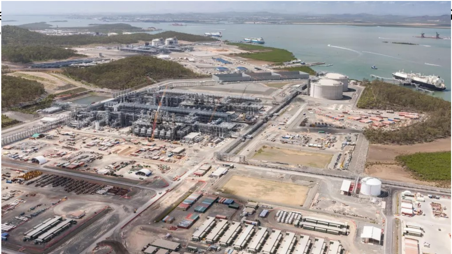
QCLNG, GLNG & APLNG on Curtis Island near Gladstone, Queensland
