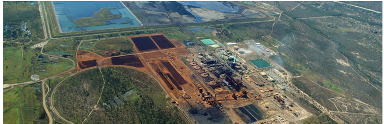
Yabulu Nickel Refinery
