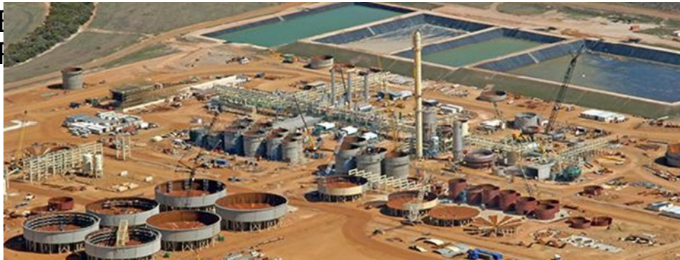
Ravensthorpe Nickel Concentrator during construction
